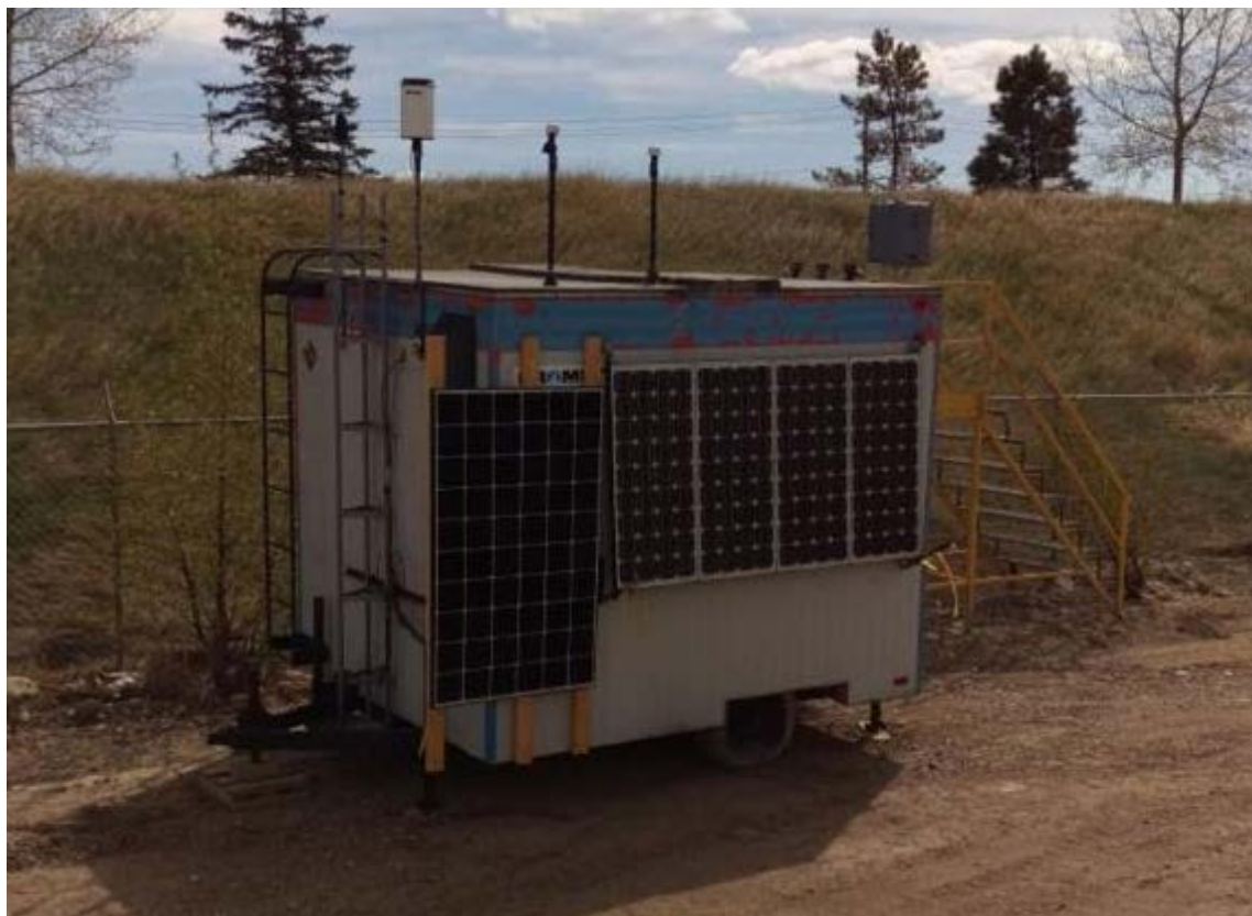
Figure A1 Picture of West Berm Station
